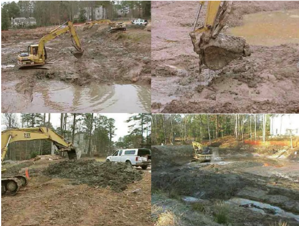
Figure AIII-28: Polymer-enhanced Mud and Sediment Removal.
