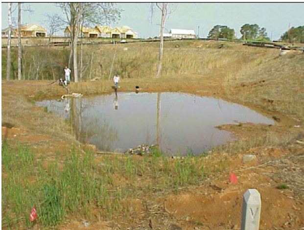
Figure AIII-2: The water was pumped out of the sediment pond.
