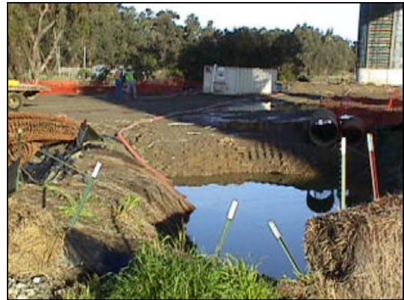
Sediment Trap (Source: http://www.mnerosion.org )
