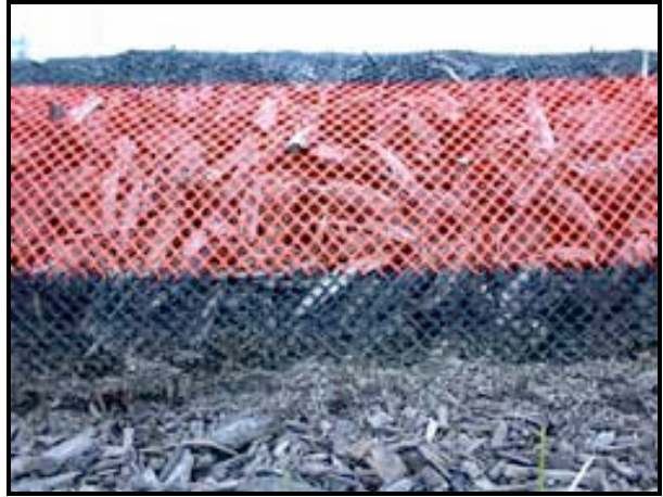
Detail of compost-filled mesh sock (Source: Filtrexx, 2006)
