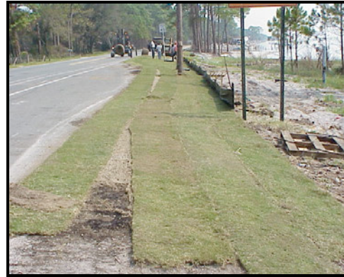
Final placement of sod
