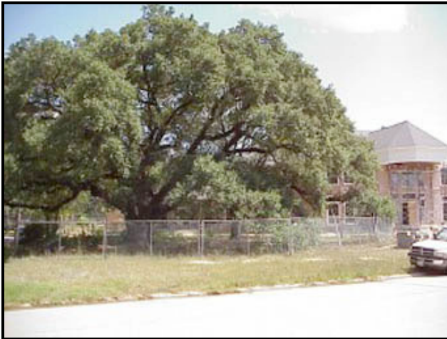
Protected tree on construction site, with fencing outside dripline (Source: Treescape, 2006)
