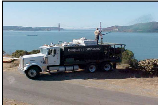
Soil binder and seed mixture applied near coastal bay (Source: SoilTac, 2006)
