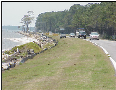
Roadway and shoulder successfully protected
