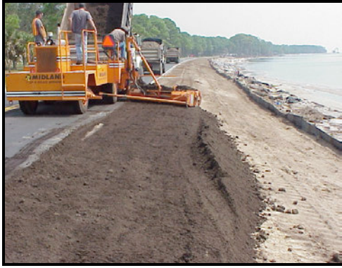
Placement of compost mulch layer
