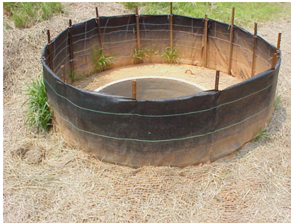
Figure AIII-12: Polymer-enhanced erosion control around drop inlet.
