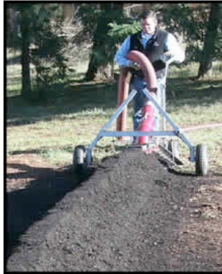
Installation of compost berm (Source: Rexus, 2006)
