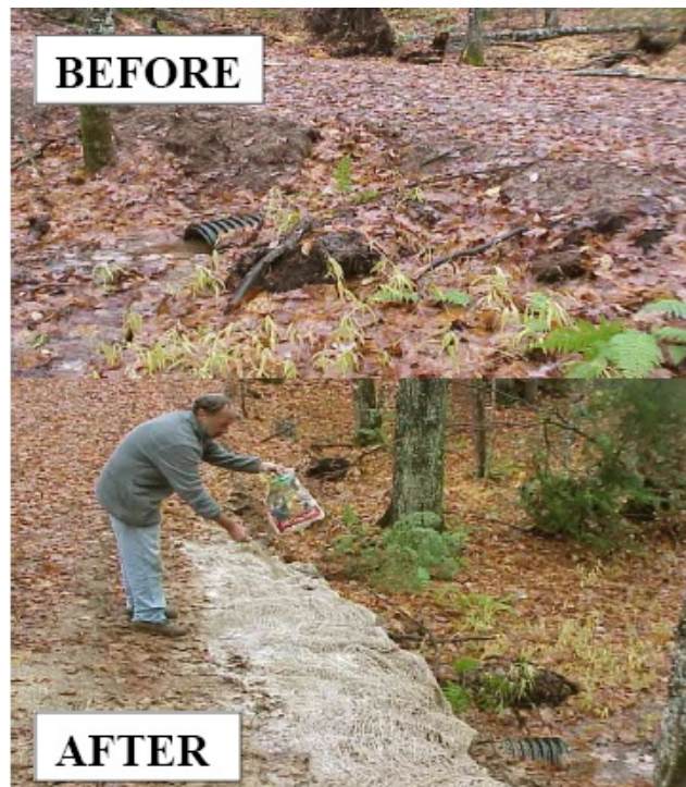
Figure AIII-10: Stream Crossing or Culvert Stabilization.
