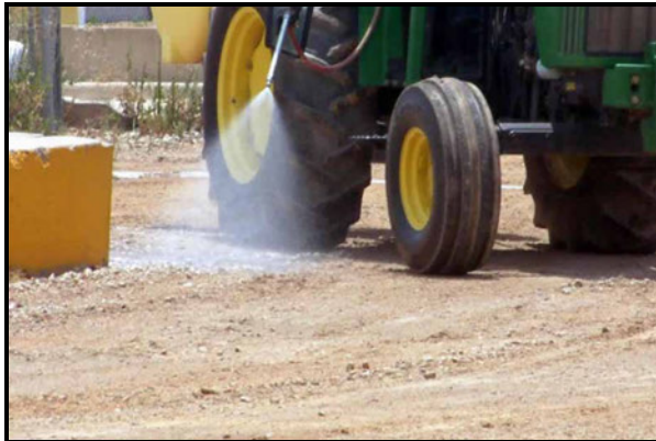
Soil tackifier applied by sprayer truck (Source: SoilTac, 2006)
